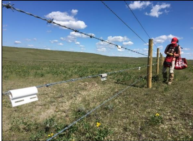
Figure 2. A volunteer installing 3" strips of vinyl siding to the top two barbed wires of a fence within Greater Sage-grouse critical habitat in Grasslands National Park, summer 2018. Photo credit: L. Gardiner/Parks Canada
