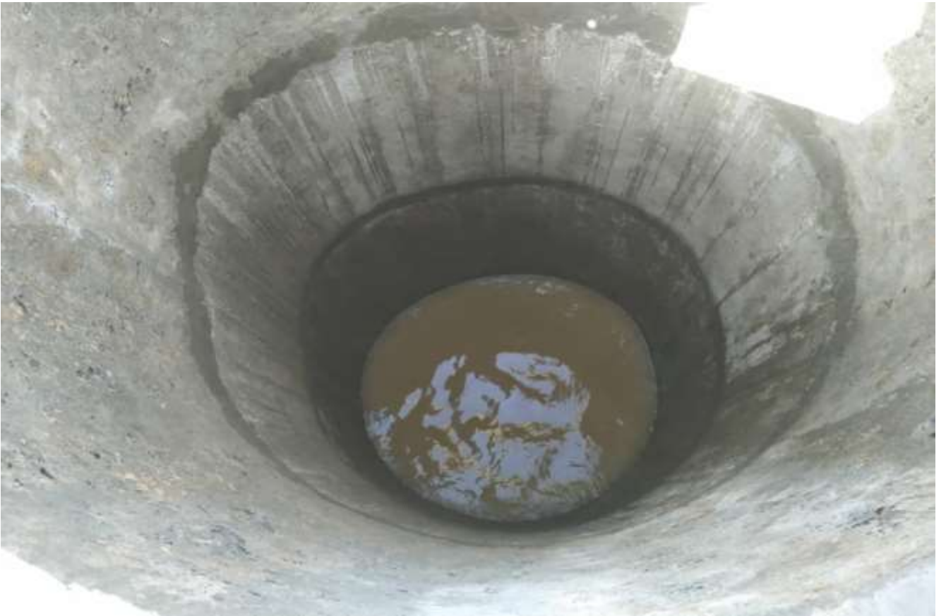
An in-depth view of this well
